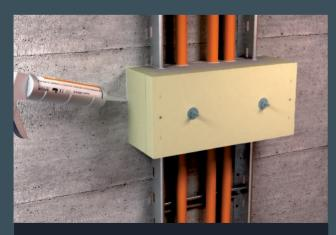
Closing of all remaining joints and sealing of the boards with  $\mbox{PYROCOAT}^{\mbox{\tiny 6}}$  ASX
