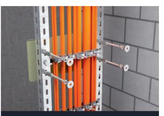
Mounting of threaded rods, locknuts and washers for fastening the housing
