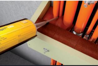
Filling with PYROPLUG<sup>®</sup> Block foam block and filling the gaps between cables with the PYROSIT<sup>®</sup> NG fire protection foam
