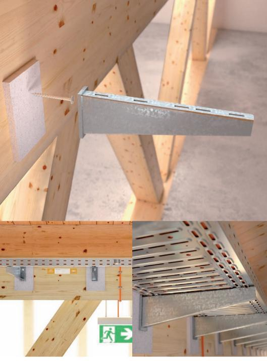
Cable route at the side on the bar in the lengthwise direction: Installation with cable tray and sloping threaded rod locking
